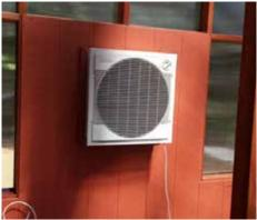
A swamp cooler will provide air circulation and humidity when connected to a water line.
