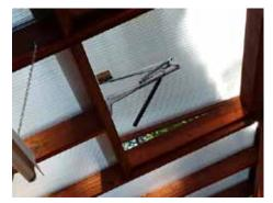
Roof vents are critical. They can be operated manually or with automatic openers. Photo by Bonnie Bradt
