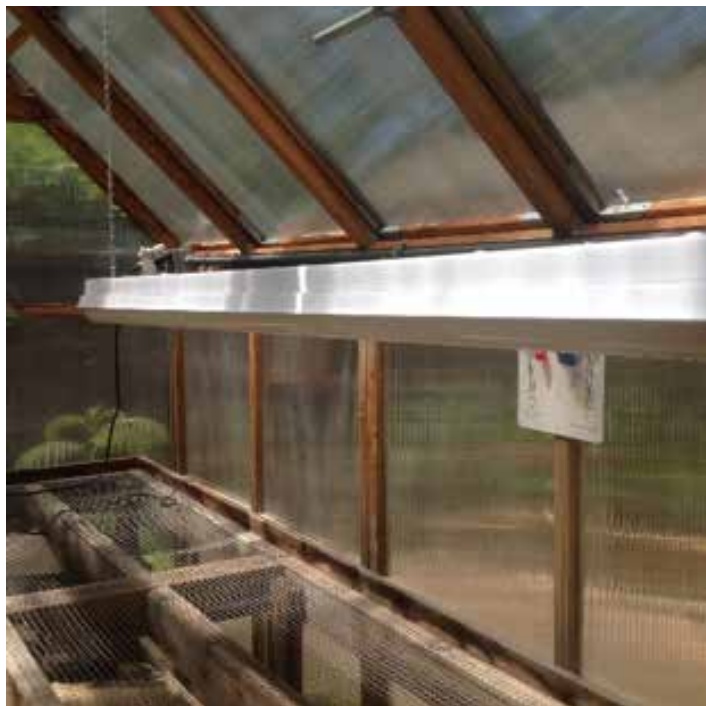
Shopligh fixtures with fluorescent bulbs can be handily used for supplemental lighting. Chains make them easy to raise and lower. Photo by Bonnie Bradt
