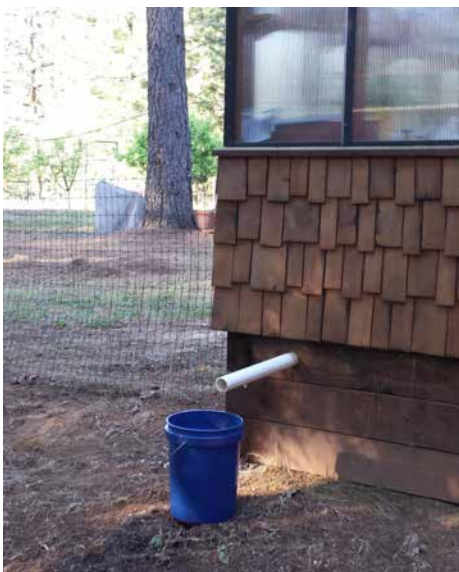
A sink (photo at right) helps water efficiently. Water can be captured and reused with the proper plumbing (above). Photos by Bonnie Bradt
