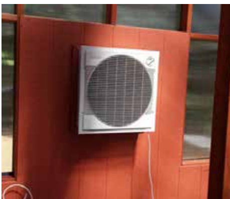
A swamp cooler will provide air circulation and humidity when connected to a water line. Photo by Bonnie Bradt
